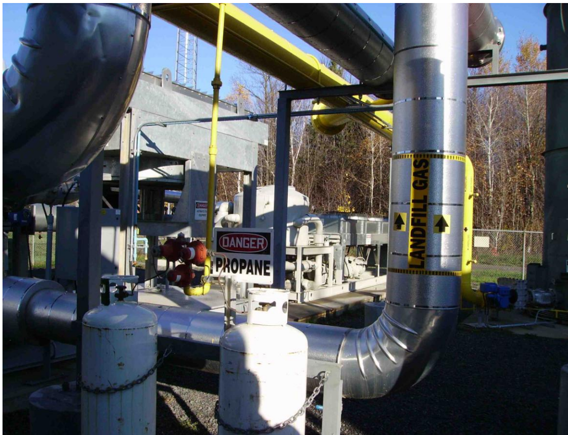
Figure 21: Landfill Gas Plant
