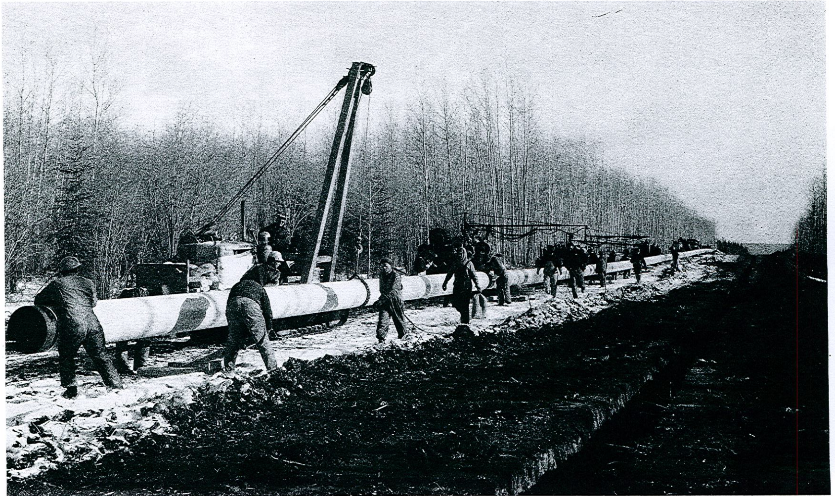
Rainbow Lake Pipeline under construction
