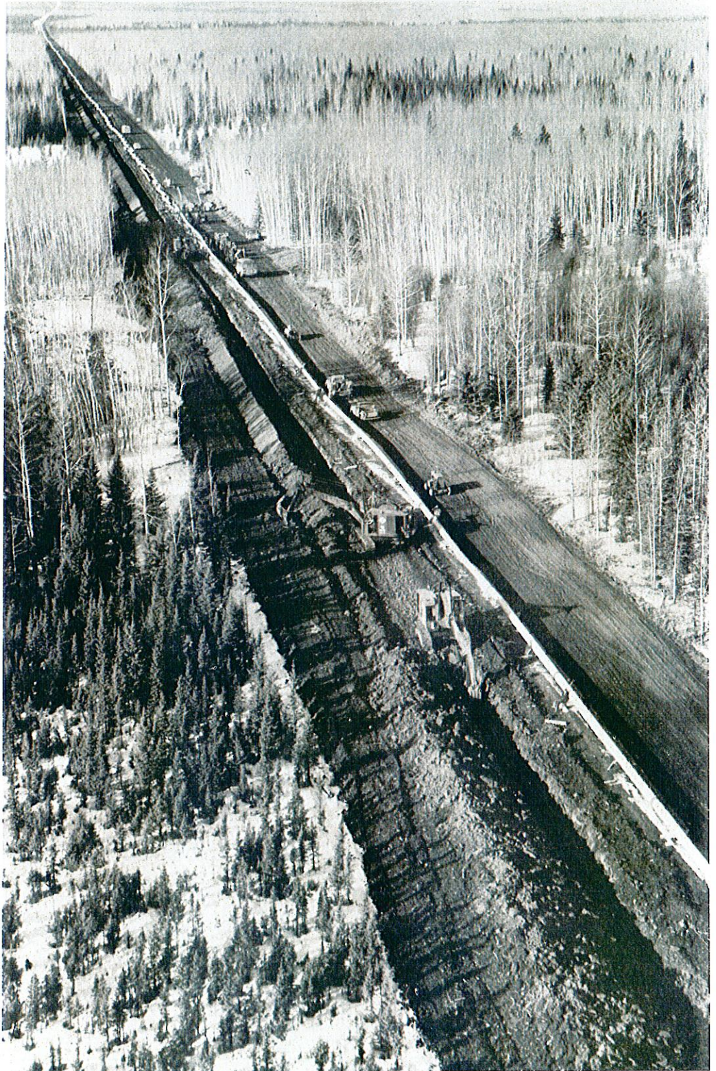
Rainbow Lake Pipeline under construction
