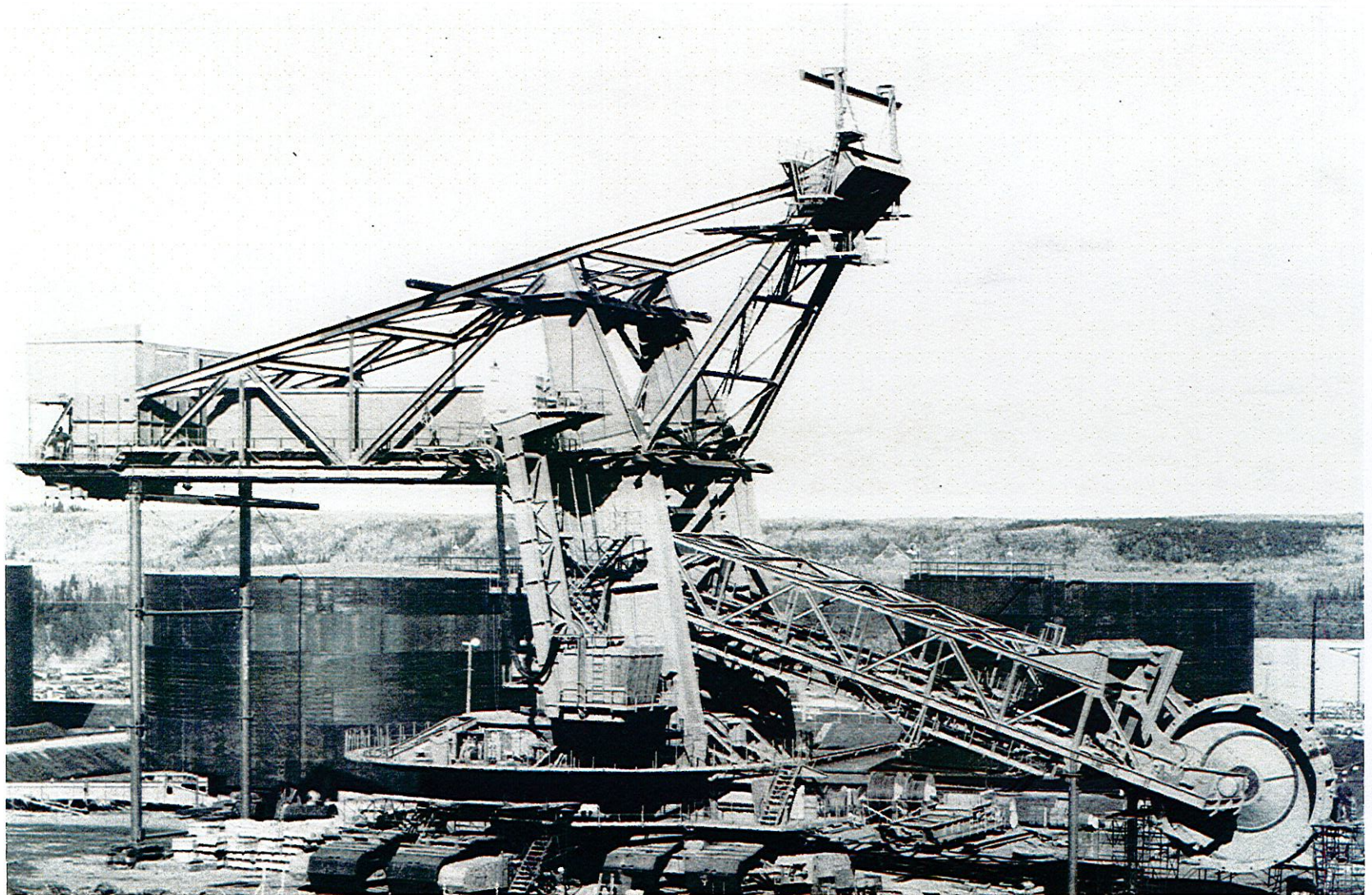
Great Canadian Oil Sands Ltd. Bucketwheel Excavator No. 1 under construction
