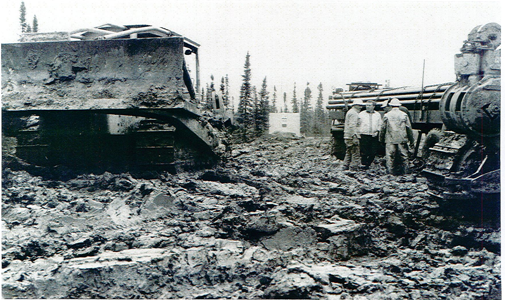
Rainbow Lake Pipeline under construction
